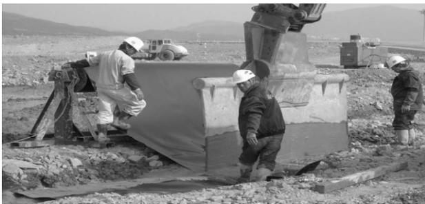
Figure 7: Installation de la membrane verticale
