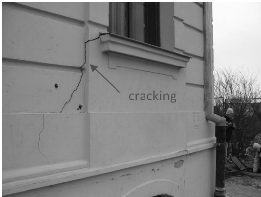
Figure 2. Crackings in facade.
