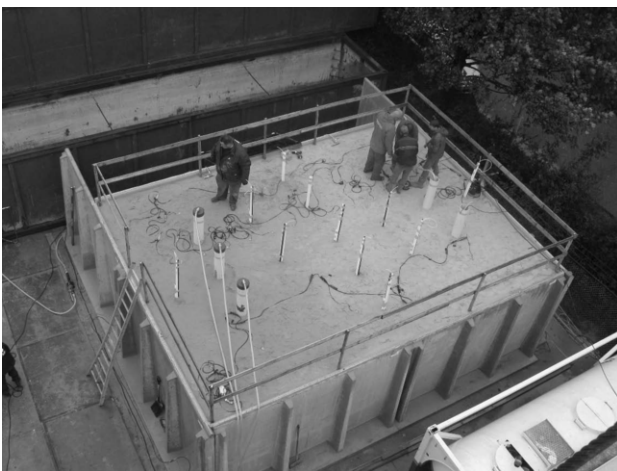
Figure 5 set-up for large scale Biogrout experiment ( 100\text{m}^3 ). Three injection wells (left) and three extraction wells (right) were used to flush liquids through the sand body.
