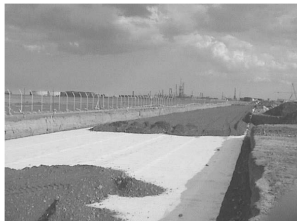
Figure 9. Installation of composite base course reinforcement
