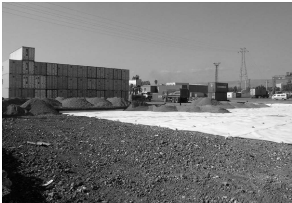
Figure 7. Installation of composite base course reinforcement
