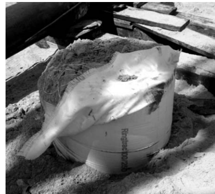
Figure 8. Recently installed sand-filled geotextile-encased column (GEC) using Ringtrac ® 100/250
