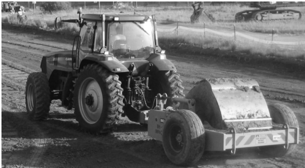
Figure 2. Impact rolling in progress.
