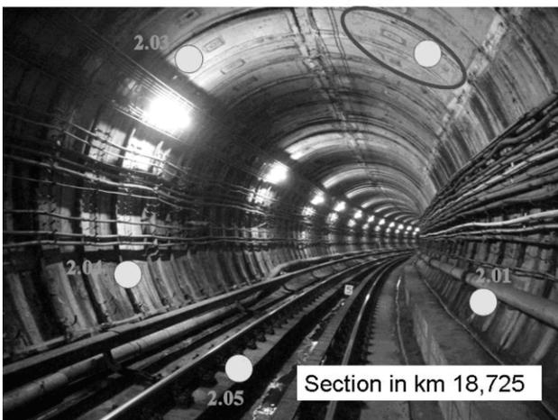
Figure 3: View of the test section 1, direction Vltavská station (tilt plates are presented by yellow circles and cracked lining segment by red ellipse where crackmeters, geophones and inclinometers are installed)
