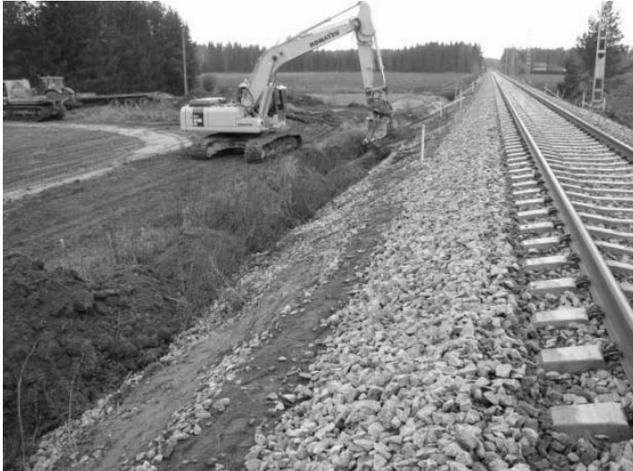
Figure 1. Shaping of the embankment sections at the Kokemäki monitoring site.
