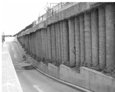
Figure 4. 7.5 m high cantilever wall at Ballycullen Rd. in service September 2007
