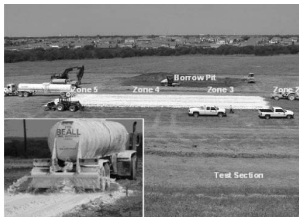
Figure 3. Construction of test sections (view from crest of dam) (Inset: Spreading of lime slurry).
