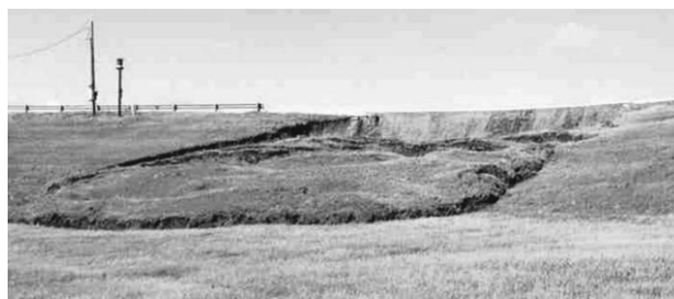
Figure 2. A typical surficial failure at Joe Pool Dam.
