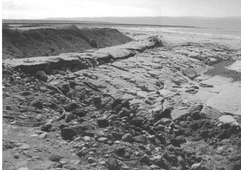
Fig. 5: Mud-wave resulting from placement of fill
