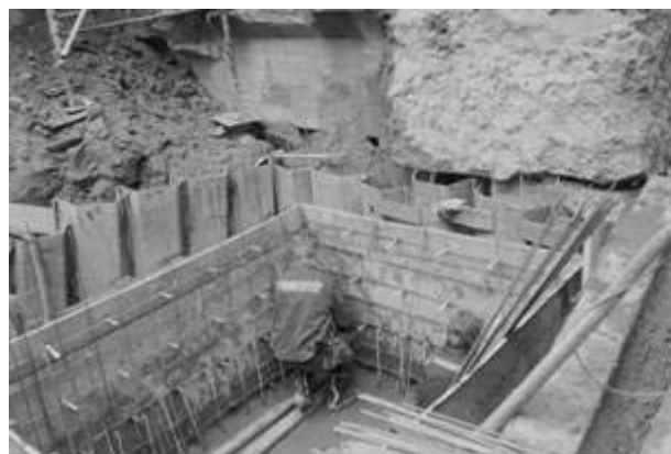
Figure 5. Elevator shaft with exposed underpinned foundation behind.
