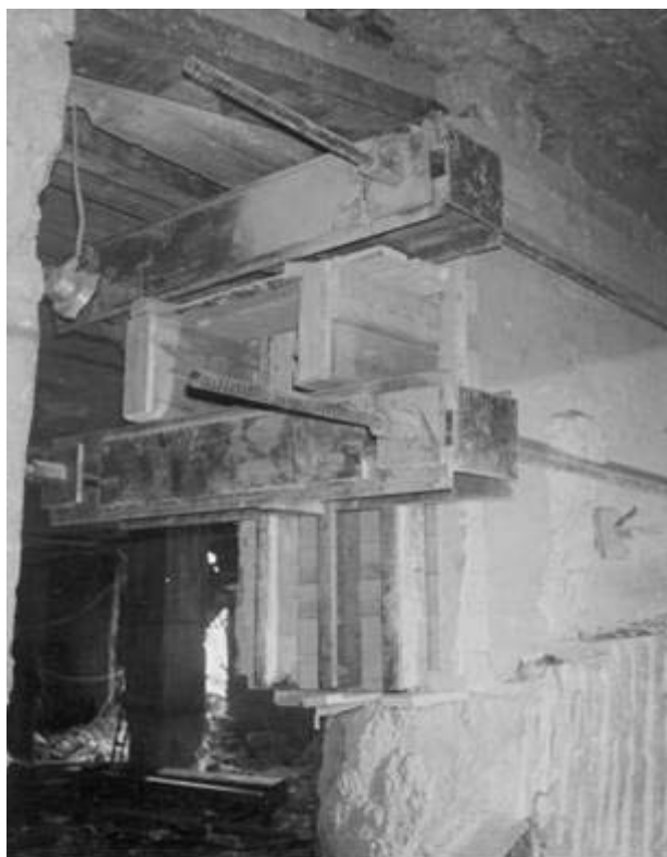
Figure 6. View of pretensioning device.
