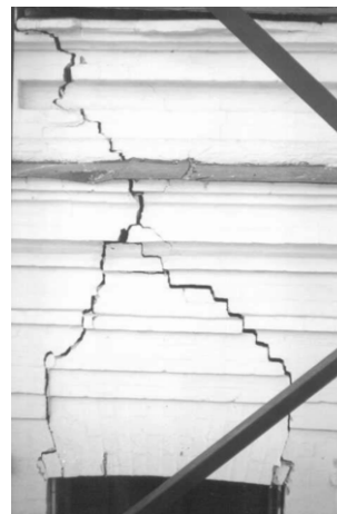
Figure 1. The failures of the MFA of Ukraine Diplomatic Academy building walls:
