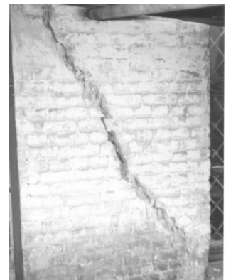
Figure 1. The failures of the MFA of Ukraine Diplomatic Academy building walls:
