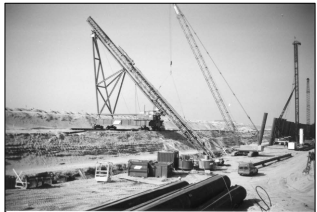
Figure 4 Pile Installation
