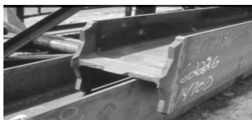
Figure 7. Steel pile with a steel tip
