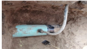
Figure 9. Actual picture of digging verification
