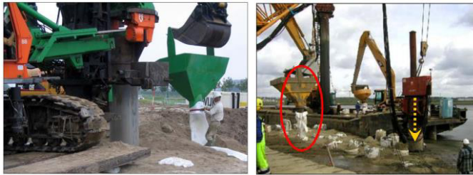
Figure 5. Installation of geotextile encasement [9]
